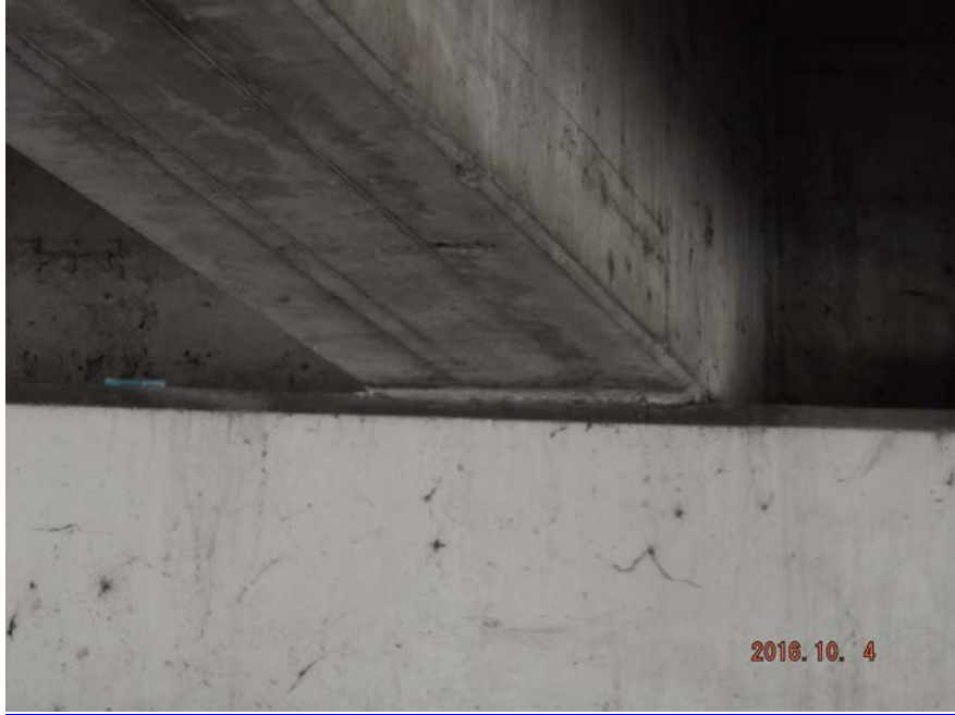
BEARINGS - ABUTMENT - ABUTMENT 1
