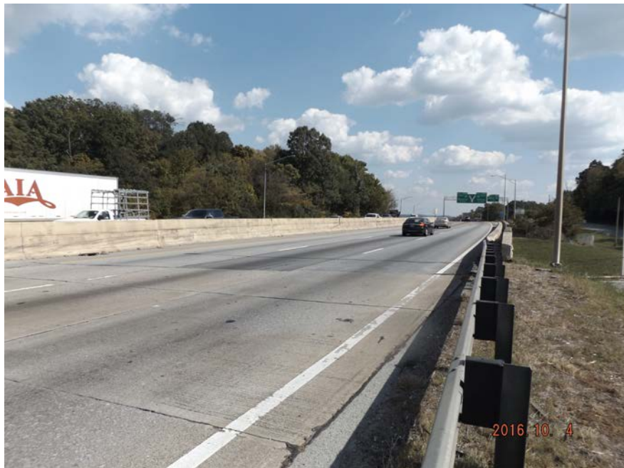
LOOKING AHEAD ON STRUCTURE
