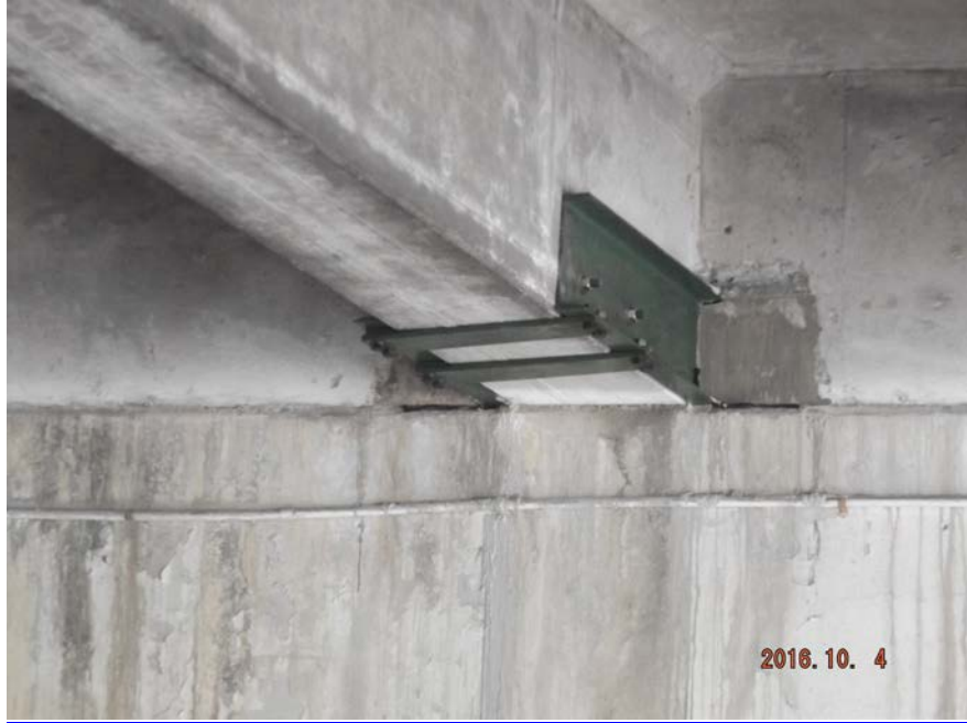
BENT 1 - NEW - REINFORCEMENTS - TYPICAL
